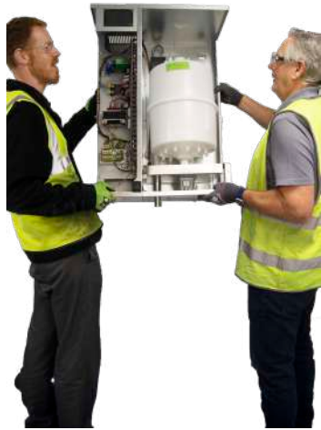
Fig 2d - Hanging the unit onto the tab inserts on the bracket
