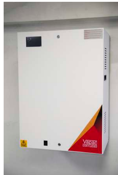
Fig 2j - Humidifier mounted with front panel locked in place
