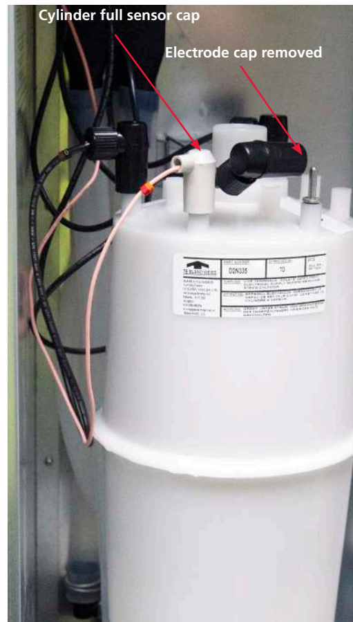
Fig 15 - steam cylinder showing electrode caps
